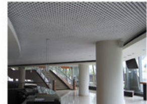
Esplanade Theatres On The Bay Lyrics Theatre Foyer 6mm thk GRG perforated ceiling
