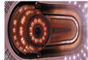
Esplanade Theatres On The Bay Concert Hall 50mm thk GRG panels forming air-con plenum
