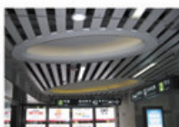
Train Station Curve Ceiling
