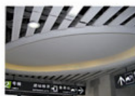
Train Station Curve Ceiling 2
